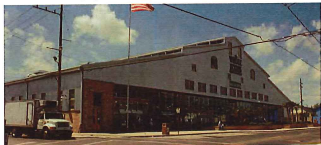
Above: The historic bus barn before rehabilitation. Below: The historic bus barn after conversion to a grocery store. A butt glazed storefront was installed in the former garage bays to retain the sense of openness.
