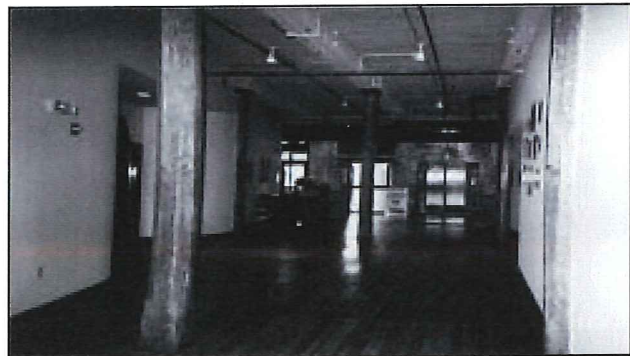
Interior after rehabilitation retains the exposed structure and finishes characteristic of the mill building with subdivision of the space for the new use.
