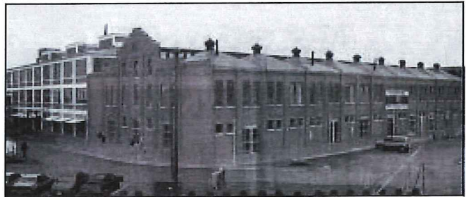
Tin can factory following rehabilitation.
