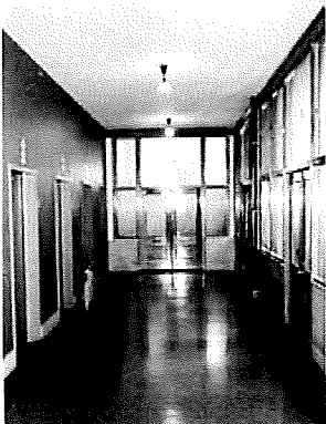
This corridor has glazed walls, oak trim, and marble wainscoting, typical of those found in the late 19th and early 20th century office buildings. Corridors such as this, displaying simple detailing, should be a priority in rehabilitation
